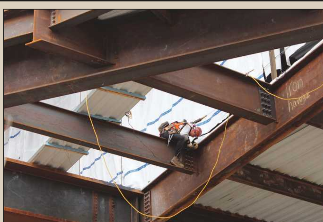
SETTING IRON at the Ford Central Campus Building in Dearborn is apprentice Mark Sawyer of Iron Workers Local 25. He's employed by Barton Malow.
